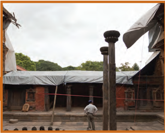
Sundari Chowk, Patan Darbar – A KVPT worker surveys the temporary tarps protecting the remainder of the fallen East Wing of Sundari Chowk from the persistent monsoon rains.
