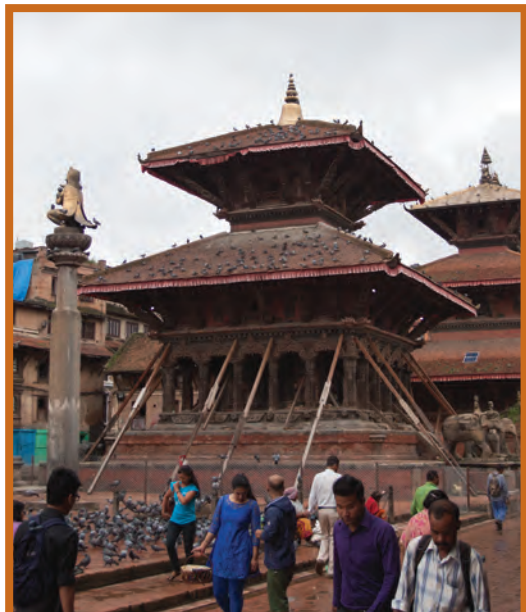
Visveshvara Temple, Patan Darbar Square, August 2015 , The main structure is still relatively intact, although the larger upper structure was torqued about the core during the earthquake. This led to severe damage to brick masonry and displacement of the timber columns and elements at the lower level of the structure. The upper levels were visibly more intact, although displaced.
