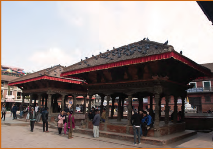
Mani Phalca (Mani Mandapa) Pavilions, Patan Darbar Square, January 2015 – Mud-brick masonry and timber structures, each supported on a grid of 16 sal wood columns. The structures were originally constructed in the 14-15th centuries, with some restorations done in the 18th century. The pavilions still included some columns thought to be original.
