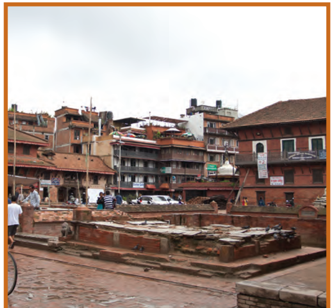
Mani Phalca Pavilions, Patan Darbar Square, August 2015 – Both Mani Phalca structures fully collapsed during the April 25, 2015 Earthquake. During cleanup and recovery, it was found that many timber columns remained fully intact during the collapses. This indicated that the structures failed at the connections between upper masonry walls and the timber columns.
