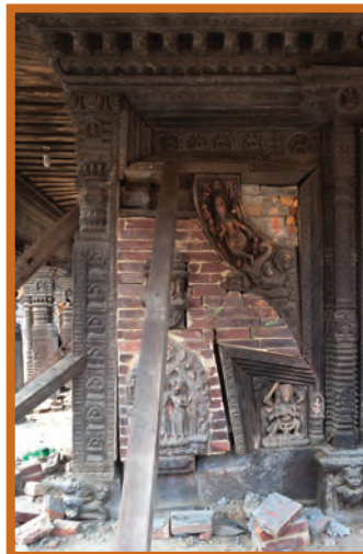
Visveshvara Temple - Eastern elevation of Visveshvara's core portal. The main load paths through the bottom floor of the temple are through the sal timber elements. The brick masonry here is, in fact, largely for aesthetics and not structural. The ability of the heavy timber elements to absorb the seismic motion and redistribute loads aided in the survival of the structure.
