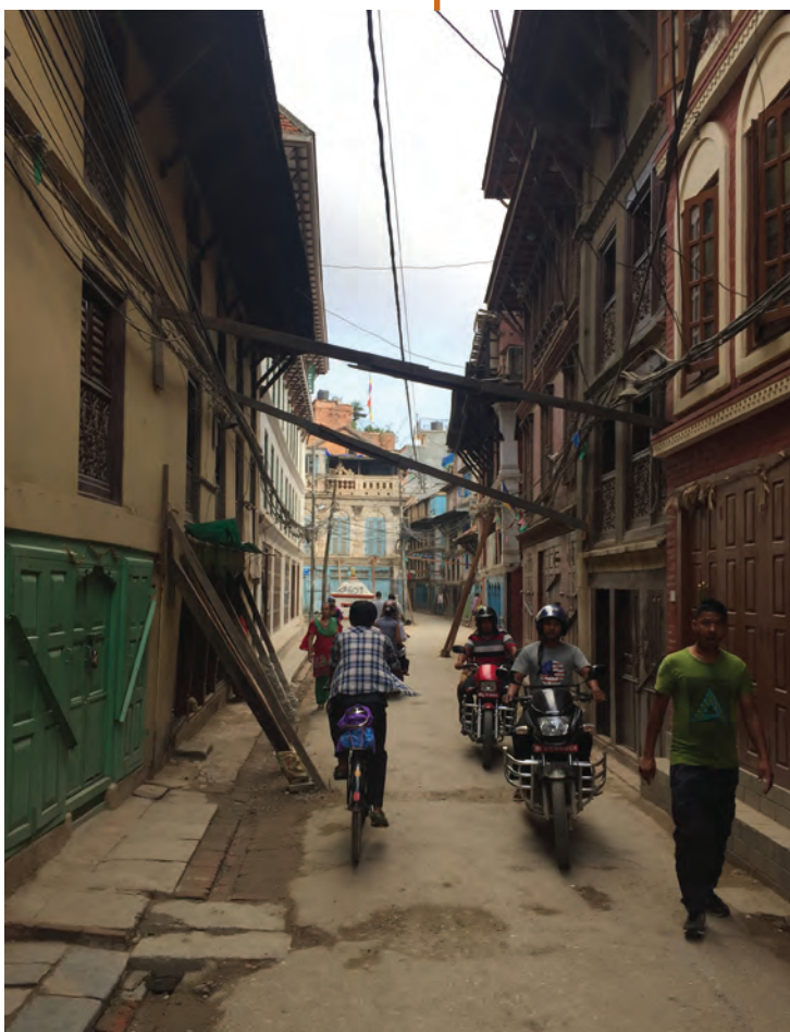
Typical temporary bracing of buildings in Patan, Nepal
