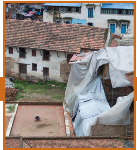
Patan Darbar near Sundari Chowk – A lone KVPT mason works to restore the brickwork of the terrace where the East Wing of Sundari Chowk, the building around the southernmost courtyard of Patan Darbar, collapsed into the garden near the Bhandarkhal water tank.
