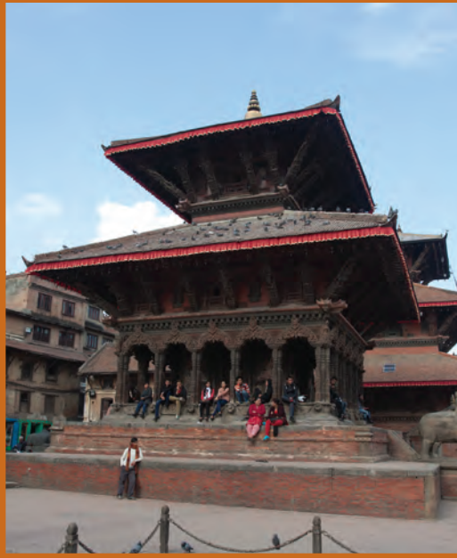
Visveshvara Temple, Patan Darbar Square, January 2015 - The Visveshvara, or Viswanath, Temple is a temple dedicated to the Hindu god Shiva and was originally constructed in the mid-17th century AD. Visveshvara is a two-tiered brick masonry and timber structure with tiled roofs laid in thick mud setting beds ranging from approximately 2" to 8" in depth. The temple's ground floor consists of a central sanctum surrounded by a carved timber and brick masonry core, surrounded by an open arcade lined with timber columns. The temple rests on a stone threshold atop a tiered plinth.
