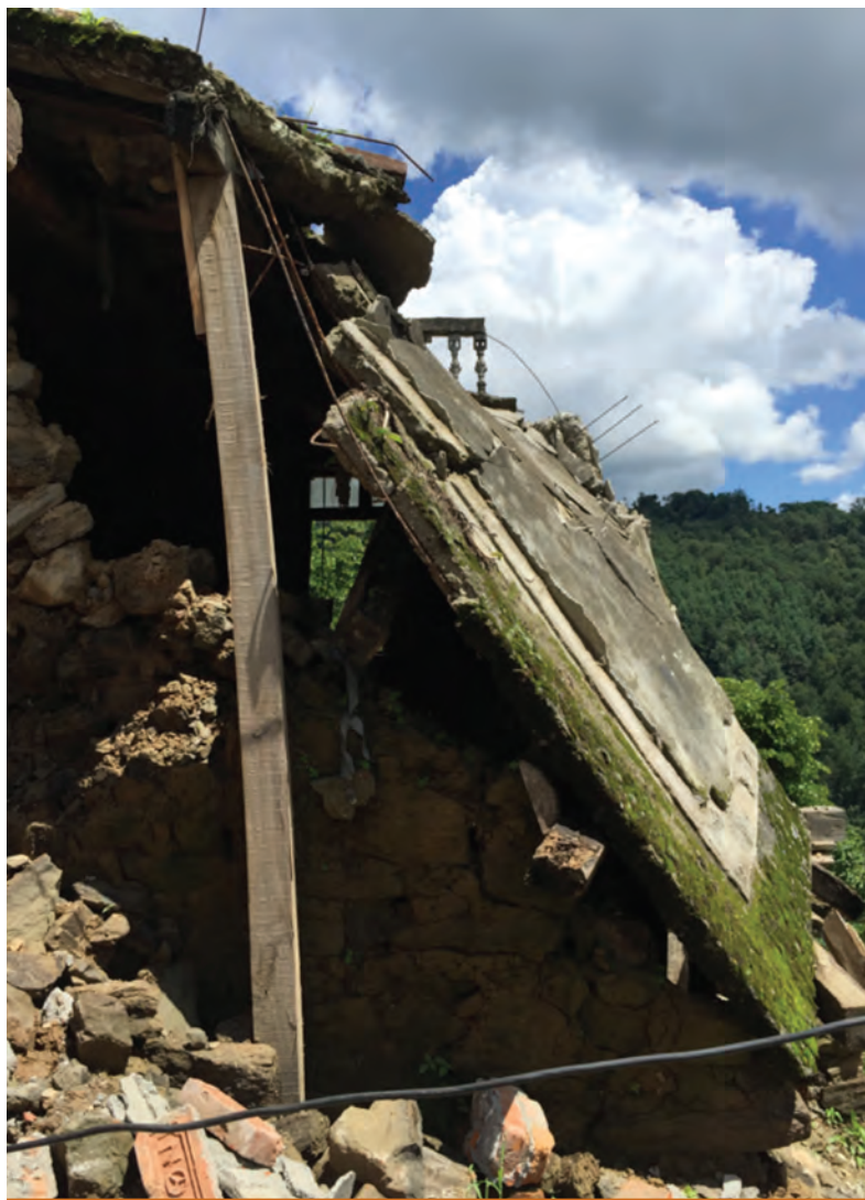
A collapsed bearing wall and floor slab at a damaged home in Nagarkot, Nepal.
