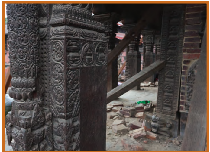
Visveshvara Temple - Detail of the main columns around the outer arcade. The timber columns shifted during the earthquake due to the movement of the brick masonry structure above.
