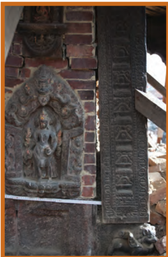
Visveshvara Temple - Column base dislodged from stone at the inner core. The original dowels and pins could not withstand the shear induced by the earthquake. Weak connections are a leading cause of displacement and failure of the historic structures in this building style.
