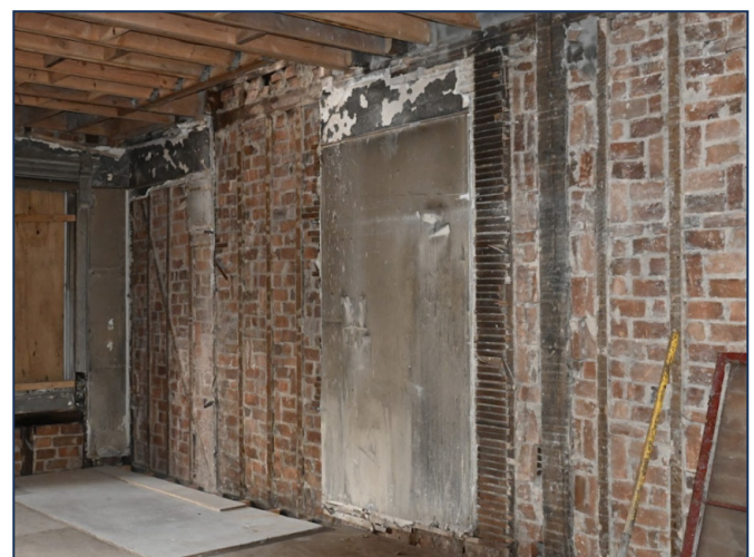
Figure 1: Nogging wall construction at townhouse under renovation in Brooklyn
