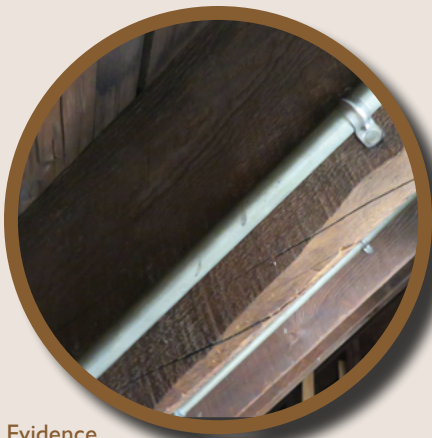
Evidence of slope of grain on a rafter as indicated by the seasoning checks
