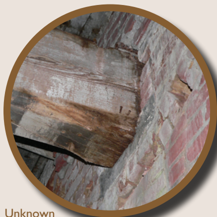
Unknown beam condition and bearing area within masonry wall
