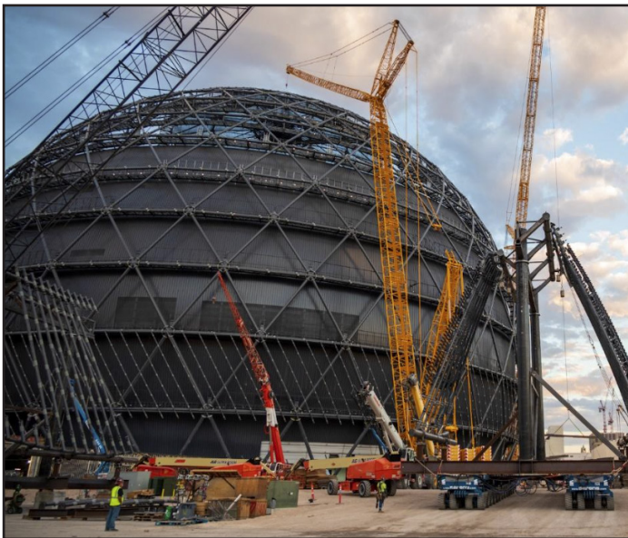
Figure 15: Setting the LED Mega Panels
