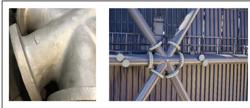
Figure 10: Erector-friendly features incorporated into the cast nodes, including "U" arrow for rapid bent assembly and metrology marks to aid in geometric control and monitoring during construction
