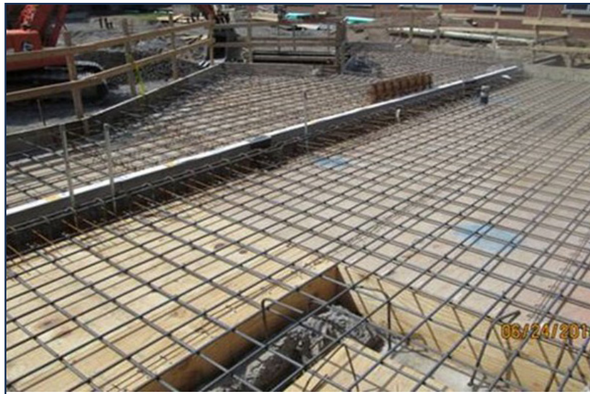
Figure 3: Concrete-to-concrete manufactured structural thermal break assembly at S.U.
