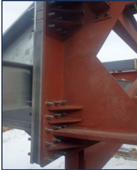
Figure 4: Large steel-to-steel manufactured structural thermal break assembly
